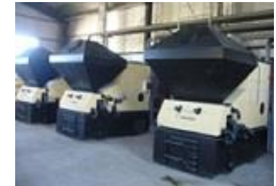
High-efficiency Heat only Boilers, Suuri-Keikaku, Mongolia
