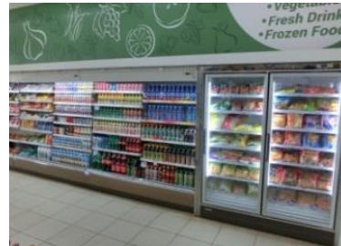
Energy saving at convenience stores, Panasonic, Indonesia
