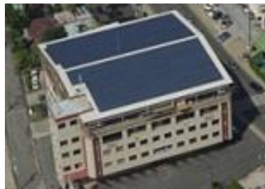
Installing solar PV system, PCKK, Palau Maldives
