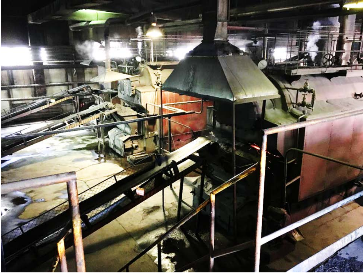
Figure 3. BEFORE: DZL (16 ton/hour steam boiler)
