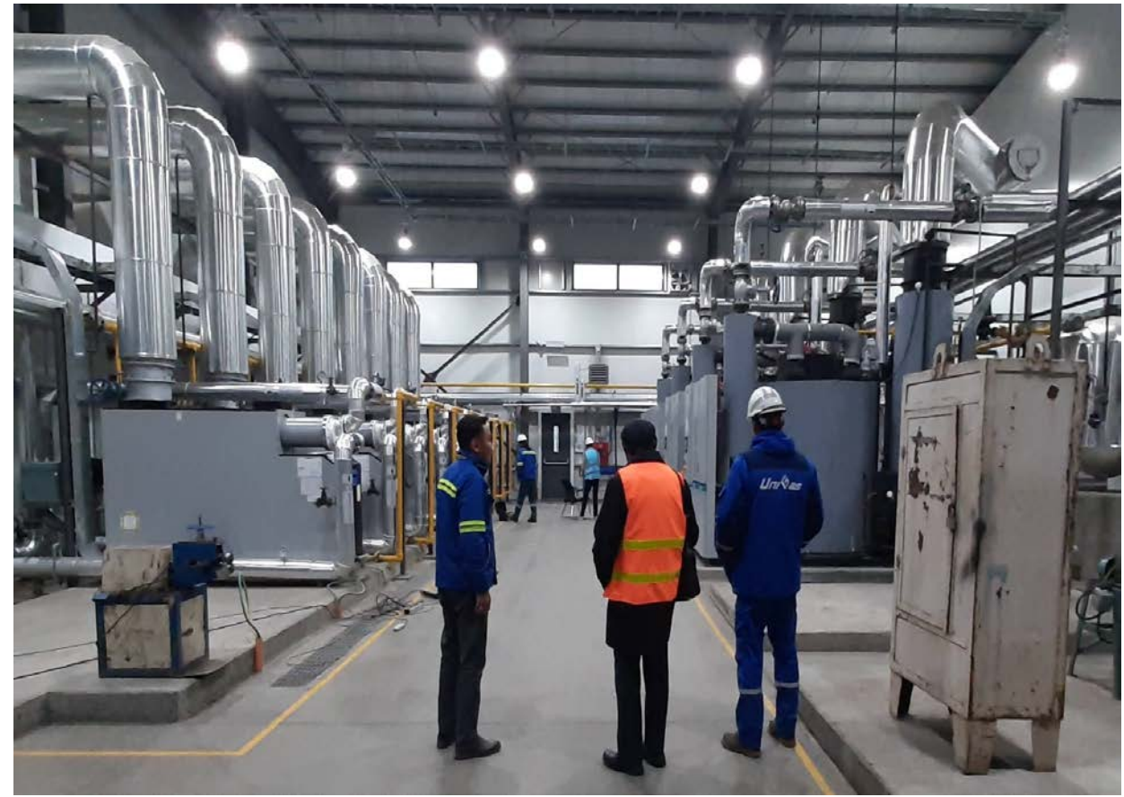
Figure 4. AFTER: DAEYEOL (4 boiler with a steam capacity of 3.4 tons), NTEC (8 boiler with a heating capacity of 0.63 GCal/h)
