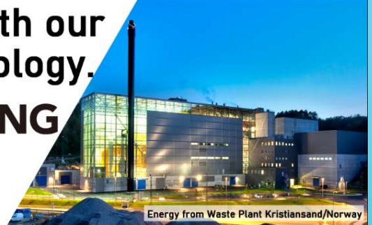
Energy from Waste Plant Kristiansand/Norway
